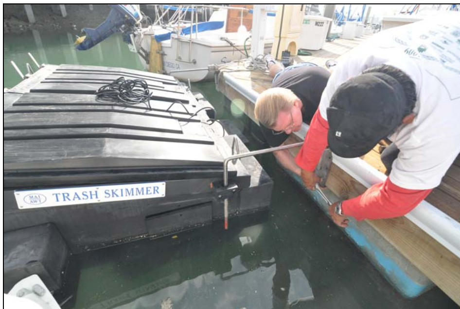
Photograph No. 6 Installation of skimmer-b
